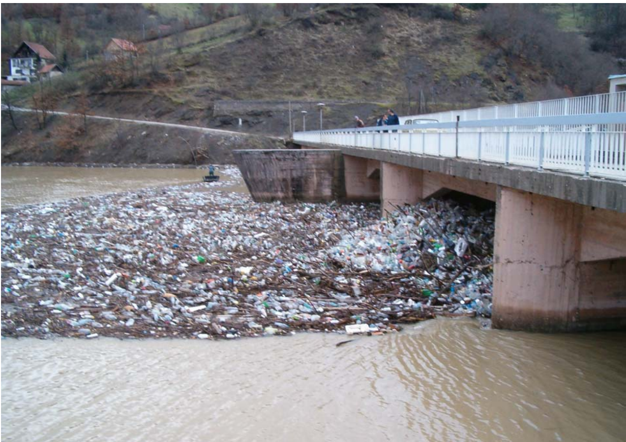
Fig.2 Hydropower plant Potpec
